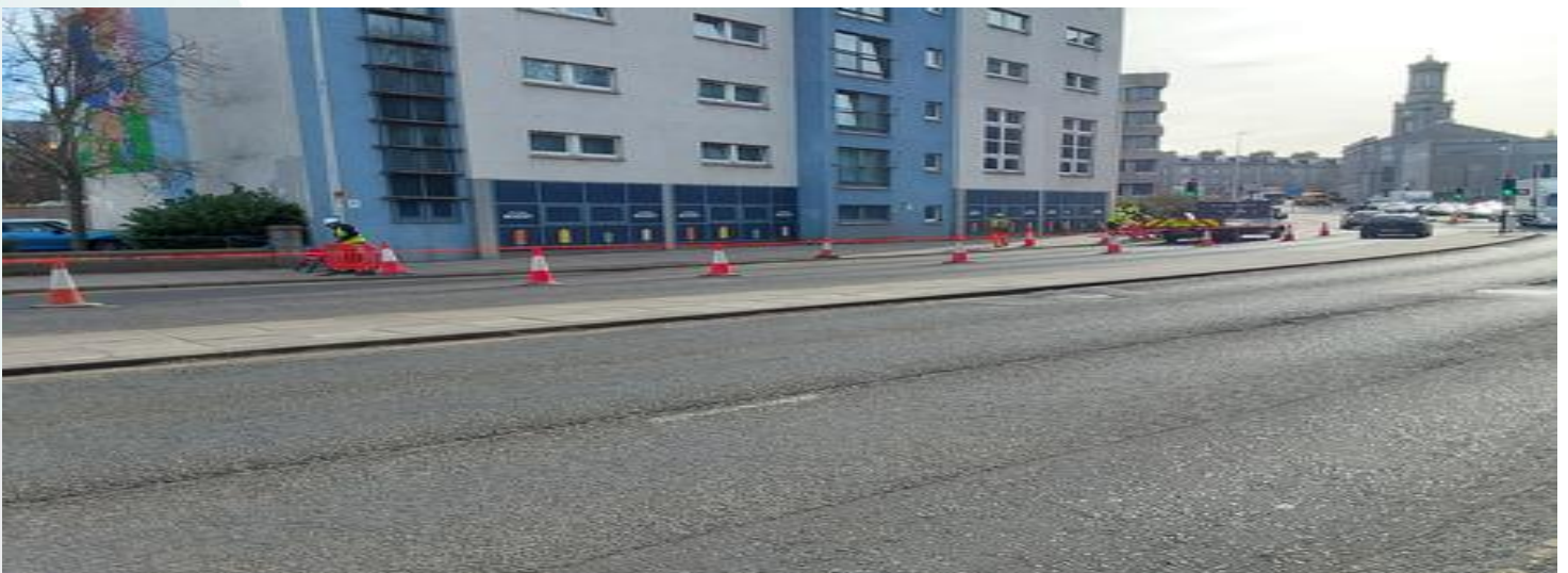
Phase 4 scaffolding lane closure and footpath restrictions.
